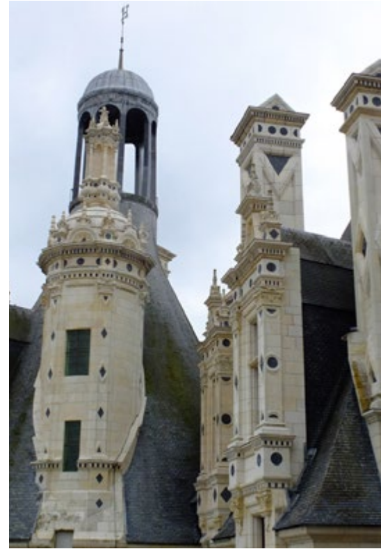
Chambord Castle, skylights and chimneys of the roof © Mission Val de Loire
