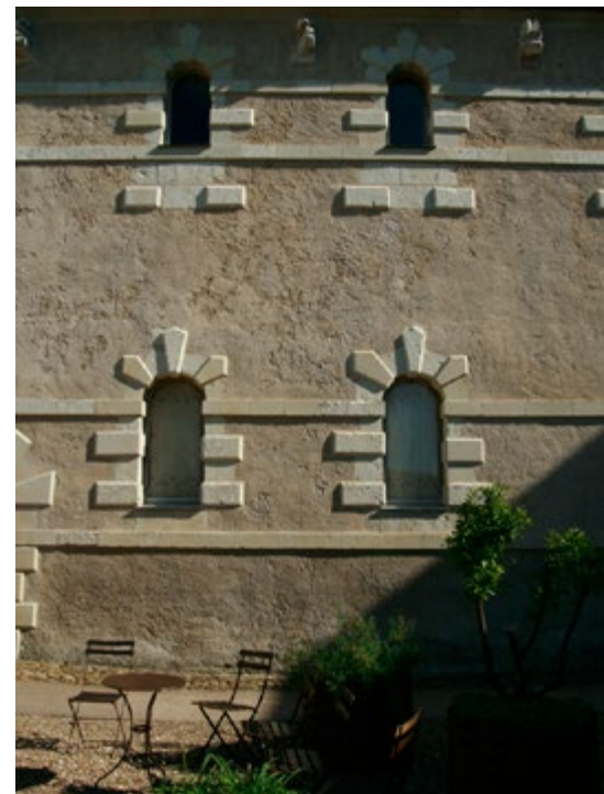
Château du Rivau, the royal stables, bossed window and door frames © Imola Gebauer
