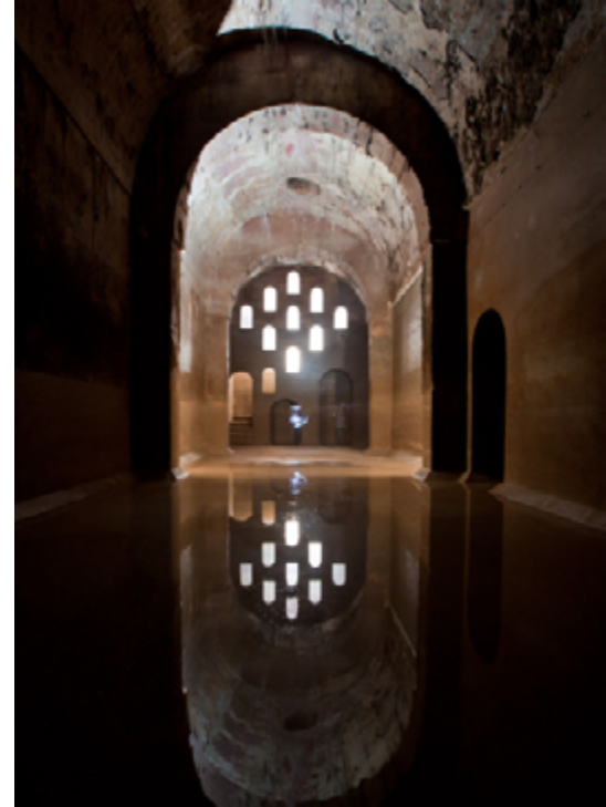
Tendilla Cistern, built for the storage and supply of water at the orders of the Governor of the Alhambra immediately after the departure of the Nasrids
