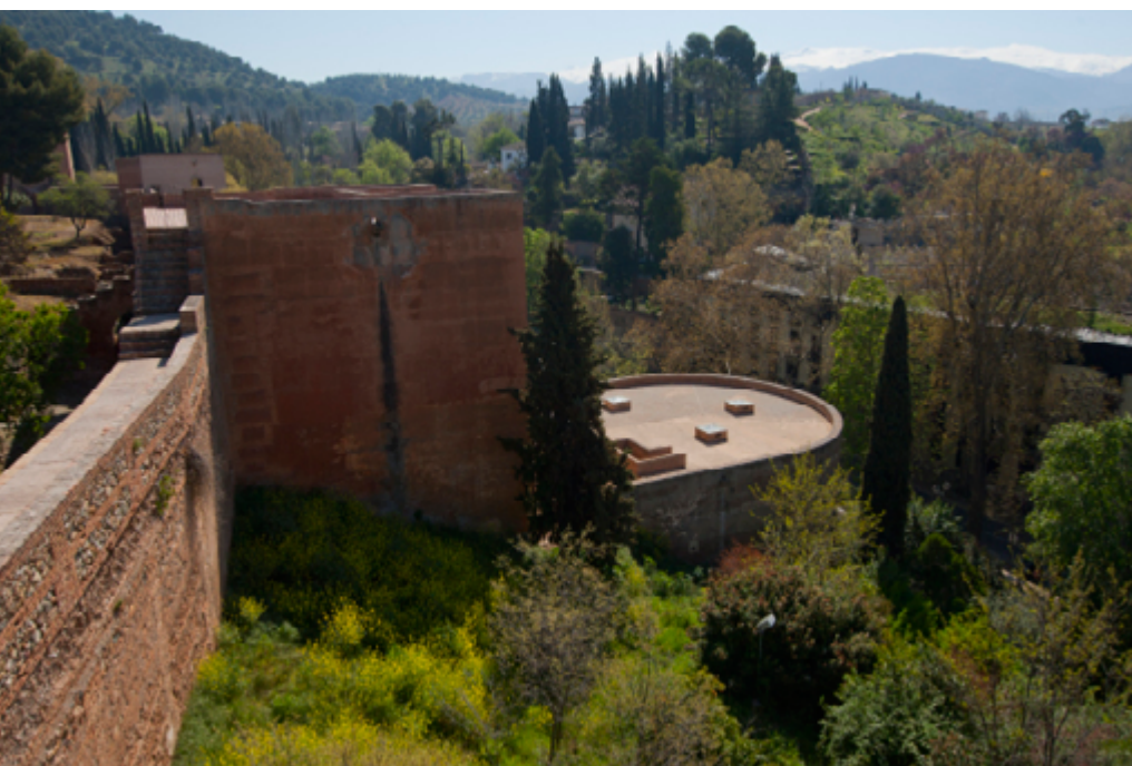
Most of the old gates and defensive towers had their bastions rebuilt with curved walls
