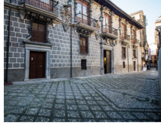
The façade of La Madraza preserves the false architectural decoration it acquired in the 18th century
