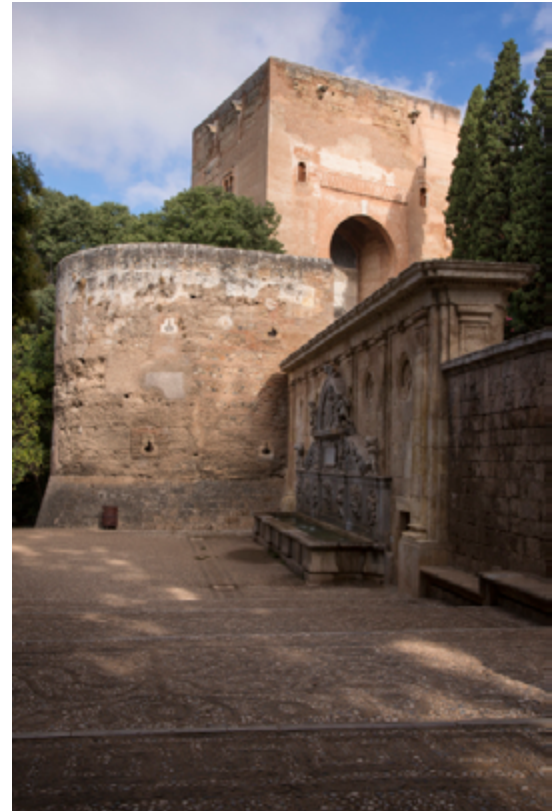
Some of the rebuilding carried out by the Castilians shortly after their arrival consisted of constructing new defences and bastions adapted to technological advances in weaponry, especially artillery
