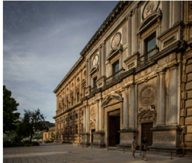
Main entrance of the palace, finished in the reign of Philip II to designs by Juan de Herrera
