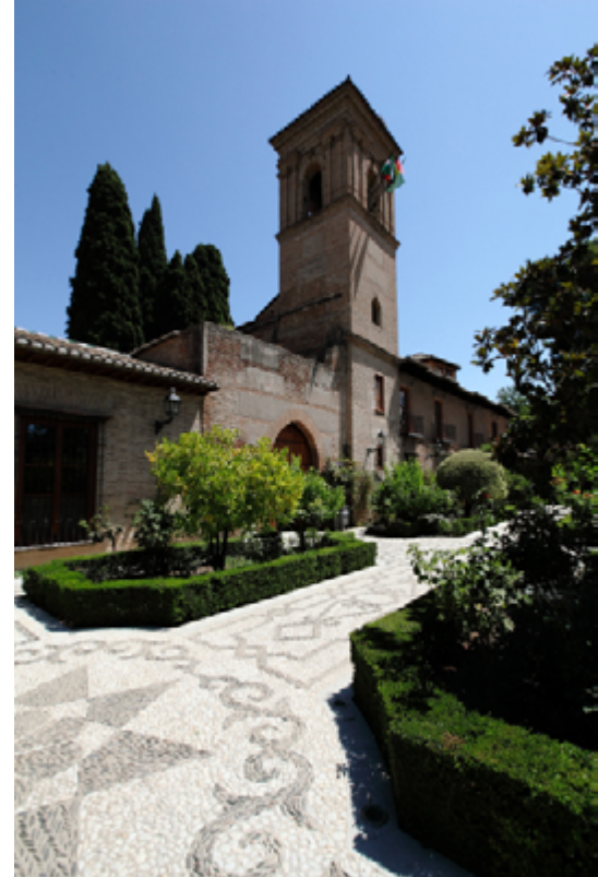
Atrium, porch and tower of the convent church
